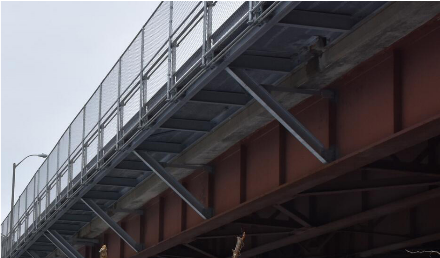
Example of a Cantilevered Sidewalk Bridge Addition
