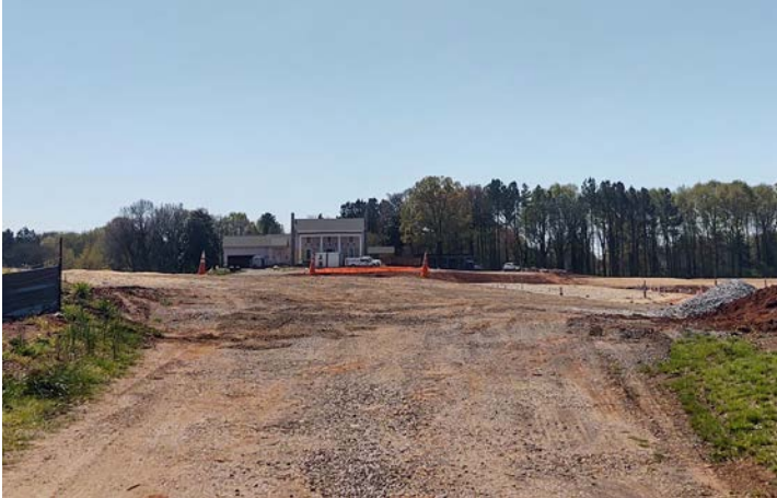
Olde Homestead Construction - Under Construction
