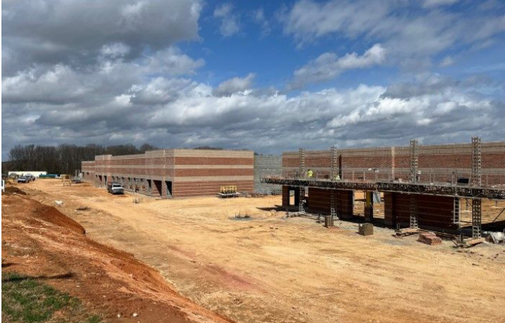
Springs Business Park - Under Construction
